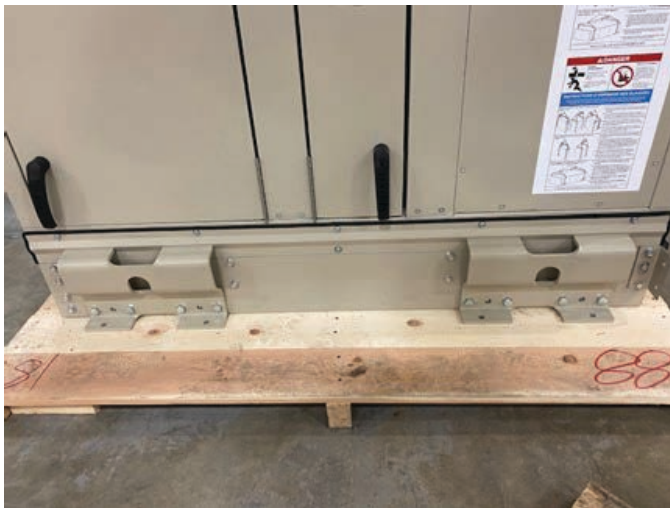
Figure 84: Lifting lugs located on base rail
