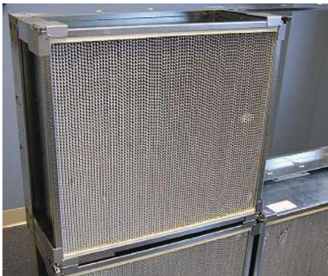
Figure 27: Properly Installed Filter Inside of the Frame
