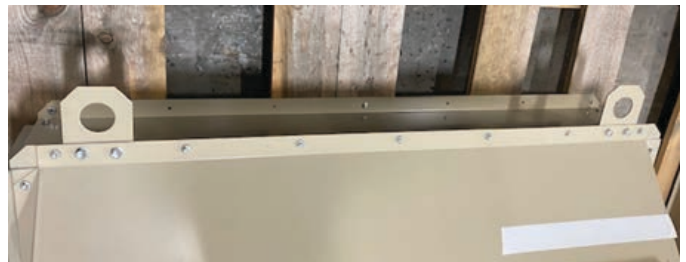
Figure 77: Bottom flange of hood screwed to unit while held in place by lifting bracket
